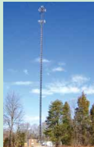
Figure 1 – A typical macrocell base station with receive antennae at the top, transmit antennae below the receive antennae, and the control system at the base.
